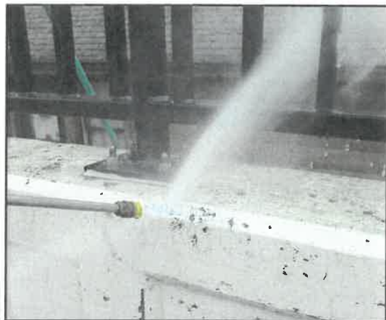
Picture 2: Pressure Wash Using Chisel Nozzle Tip
