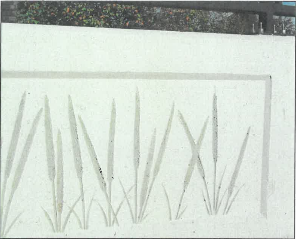
Picture 3: Painted Parapet
