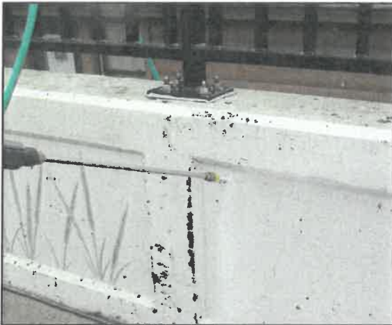
Picture 1: Pressure Washing Parapet
